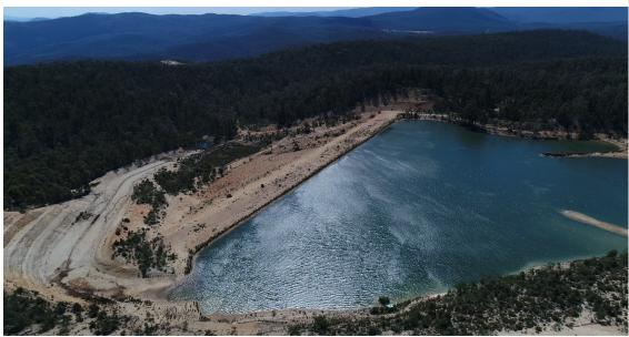
Stockman Project - Work Plan approval will permit Round Oak Minerals to double the height of the dam wall, increasing the dam surface area by almost four-fold, in order to store an additional seven million tonnes of mine waste.
