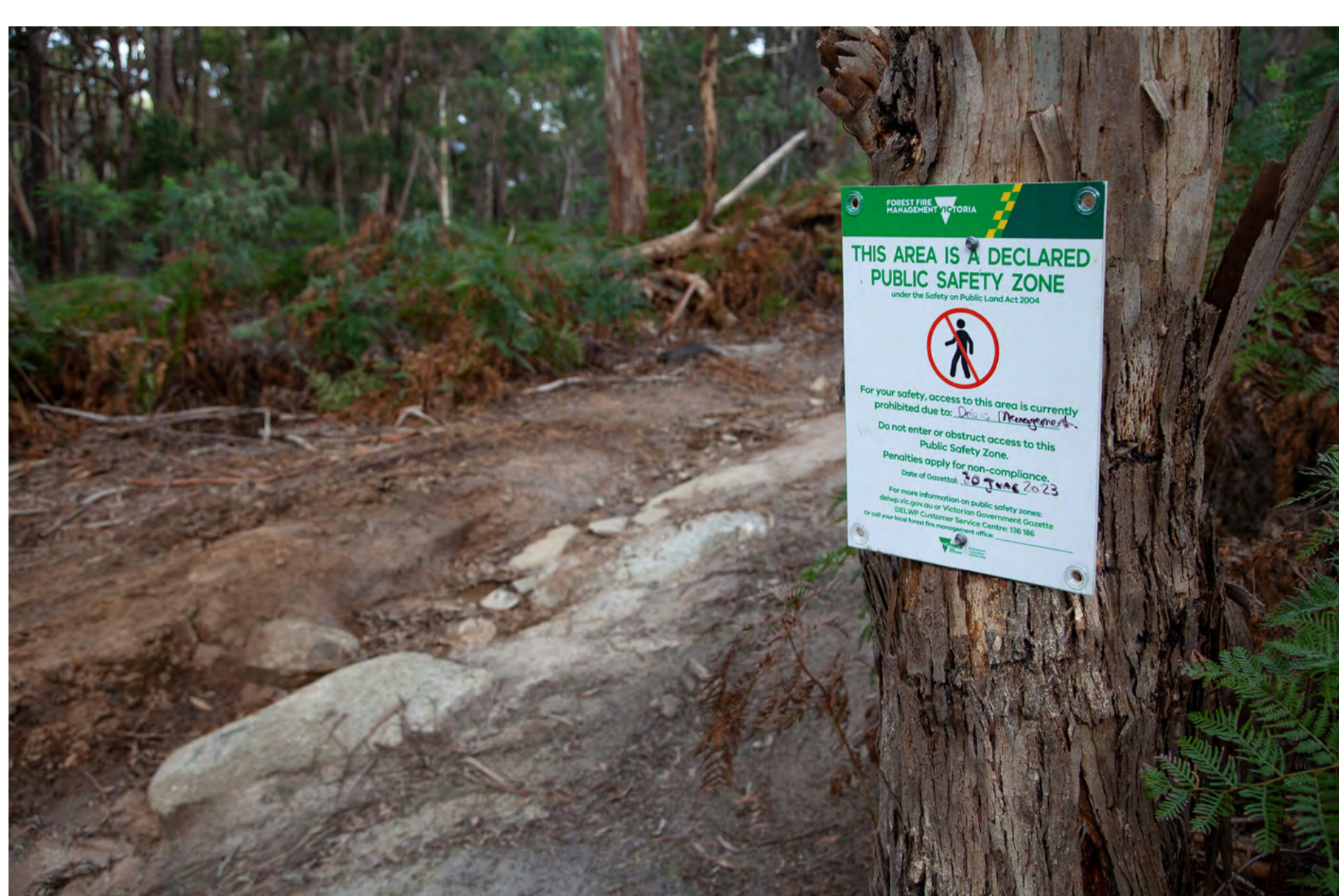
Heavy erosion in Cobaw in January 2023, with a safety zone sign from the future (Ben Gill)
