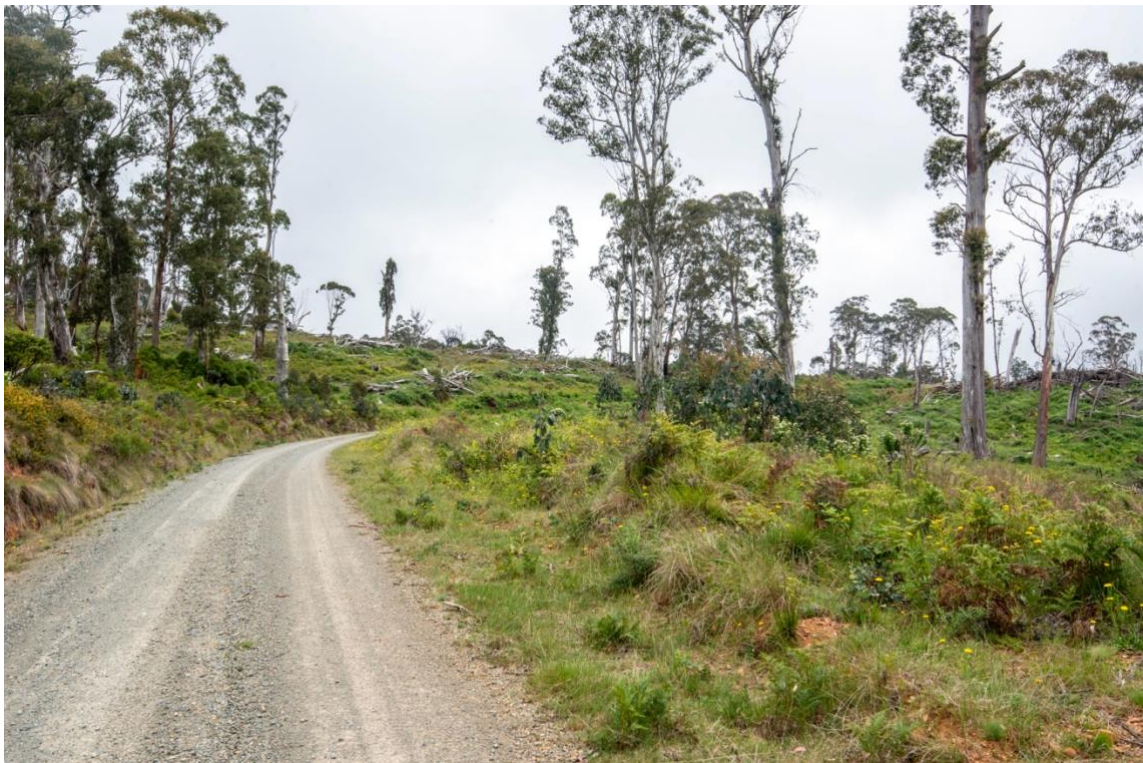
WP 318 Mt Delusion Road - Logged 2021/22. Pic: L. Roberts, 11 December 2023
